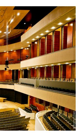
The acoustics of the Sibelius Hall in Lahti in Finland, which were designed by the legendary acoustic designer Russell Johnson, are world class. The side walls of the over 1299-seat concert hall are made of veneered wooden shells filled with sand, which ensure optimum resonance.
