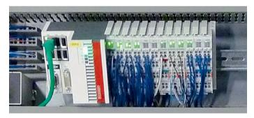
A high-performance and very compact control system was implemented using the CX5010 Embedded PC and EtherCAT Terminals.
